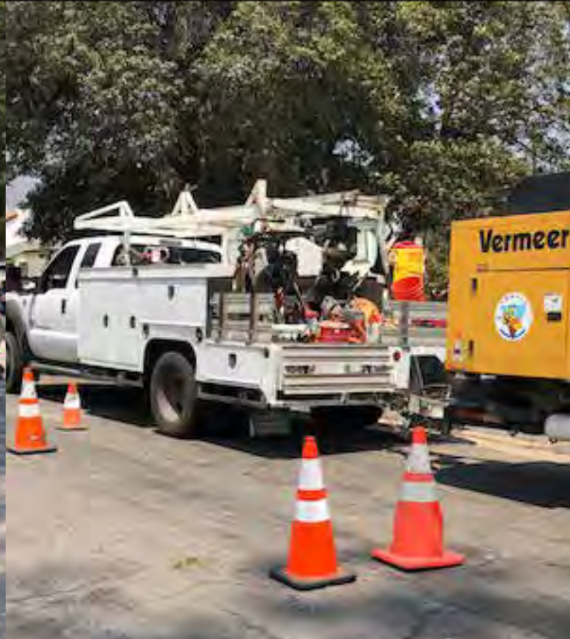
The City of Santa Paula - Public Works Department: Just another day in the office! The team works diligently to repair a 2-inch water main leak on the 600 block of N. Mill St., utilizing a jackhammer, vacuum truck, and backhoe.
