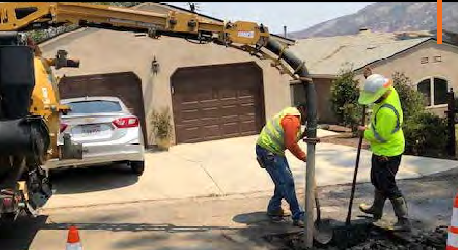
The City of Santa Paula - Public Works Department: Just another day in the office! The team works diligently to repair a 2-inch water main leak on the 600 block of N. Mill St., utilizing a jackhammer, vacuum truck, and backhoe.
