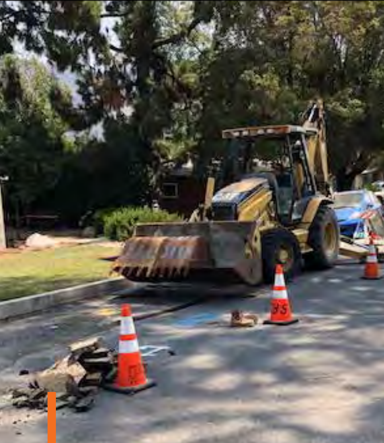
The City of Santa Paula - Public Works Department: Just another day in the office! The team works diligently to repair a 2-inch water main leak on the 600 block of N. Mill St., utilizing a jackhammer, vacuum truck, and backhoe.
